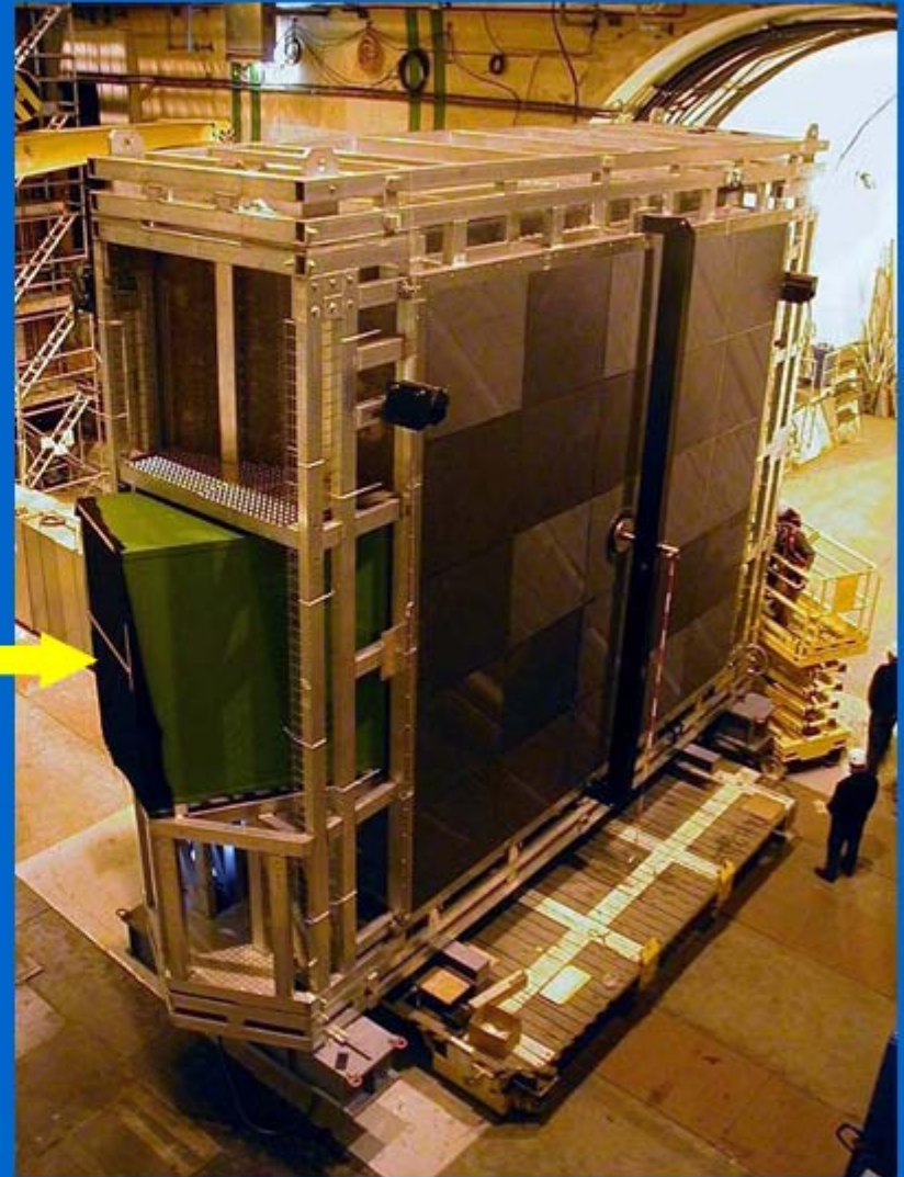
RICH2 being installed in LHCb underground cavern
